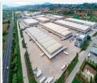
Centro Logistico Orlando Marconi Montepandone, Italy
