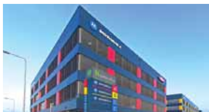
2 Green Office, 80, 80A, 82 and 84 Czerwone Maki Street, Kraków
