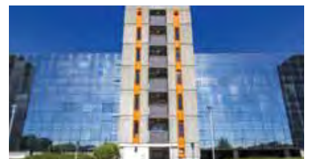
4 Building F7-F11, Milan
