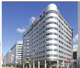
Central Plaza Rotterdam, The Netherlands
