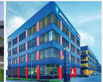
Green Office Kraków, Poland
