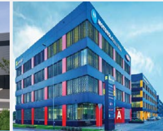
Green Office Kraków, Poland
