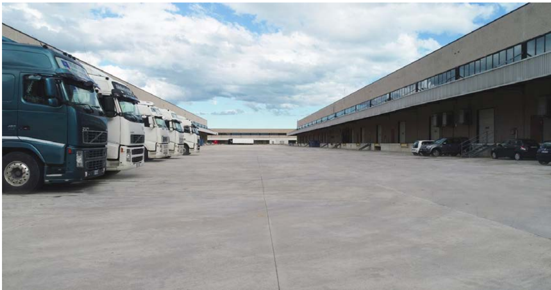
One of the Asset's warehouses and loading areas
