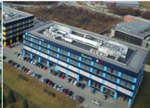
Green Office (Kraków, Poland)
