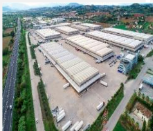
Centro Logistico Orlando Marconi Montepandone, Italy
