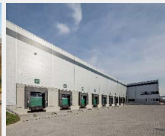
Nove Mesto ONE Industrial Park II SK Kočovce, Slovakia
