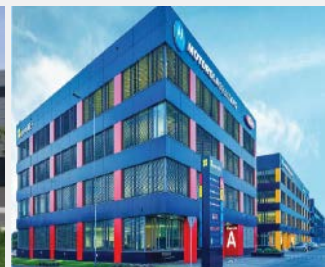
Green Office Kraków, Poland
