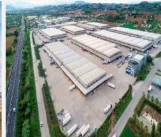
Centro Logistico Orlando Marconi Montepandone, Italy
