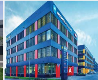
Green Office Kraków, Poland
