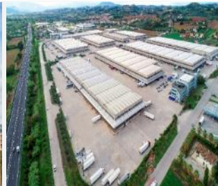
Centro Logistico Orlando Marconi Montepandone, Italy
