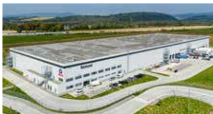
2 Nove Mesto ONE Industrial Park I, Beckov
