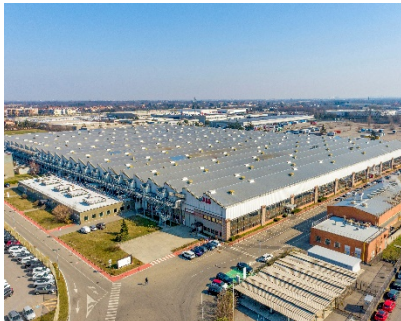
ABB Industrial Site Vittuone, Milan, Italy
