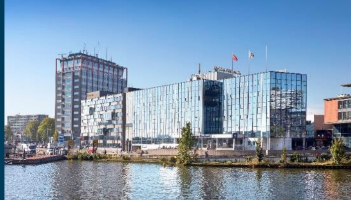
Potential redevelopment De Ruyterkade 5
