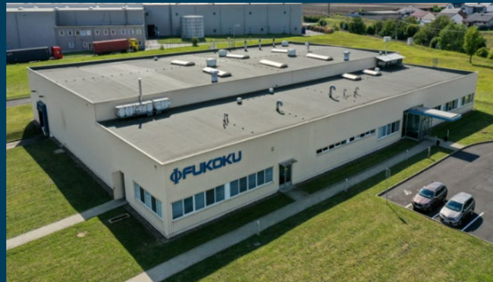
Commenced building extension development Lovosice ONE Industrial Park I
