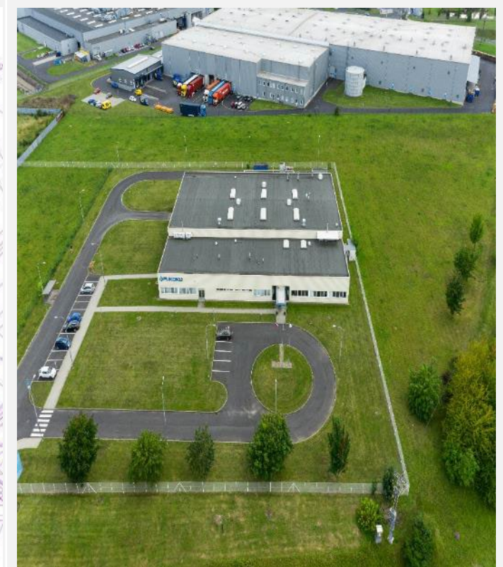
Lovosice ONE Industrial Park I and II: existing buildings – actual aerial view
