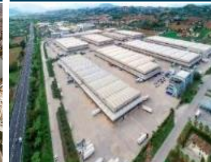
Centro Logistico Orlando Marconi (CLOM) Monteprandone, Italy
