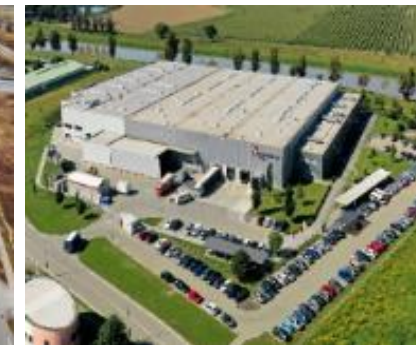
Moravia Industrial Park Uherské Hradiště, The Czech Republic
