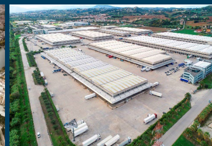
Centro Logistico Orlando Marconi (CLOM) Montepandone, Italy
