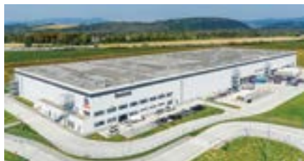
1 Nove Mesto ONE Industrial Park I, Beckov
